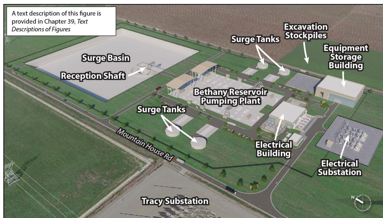
21 22 Figure 3-31. Bethany Reservoir Pumping Plant and Surge Basin
