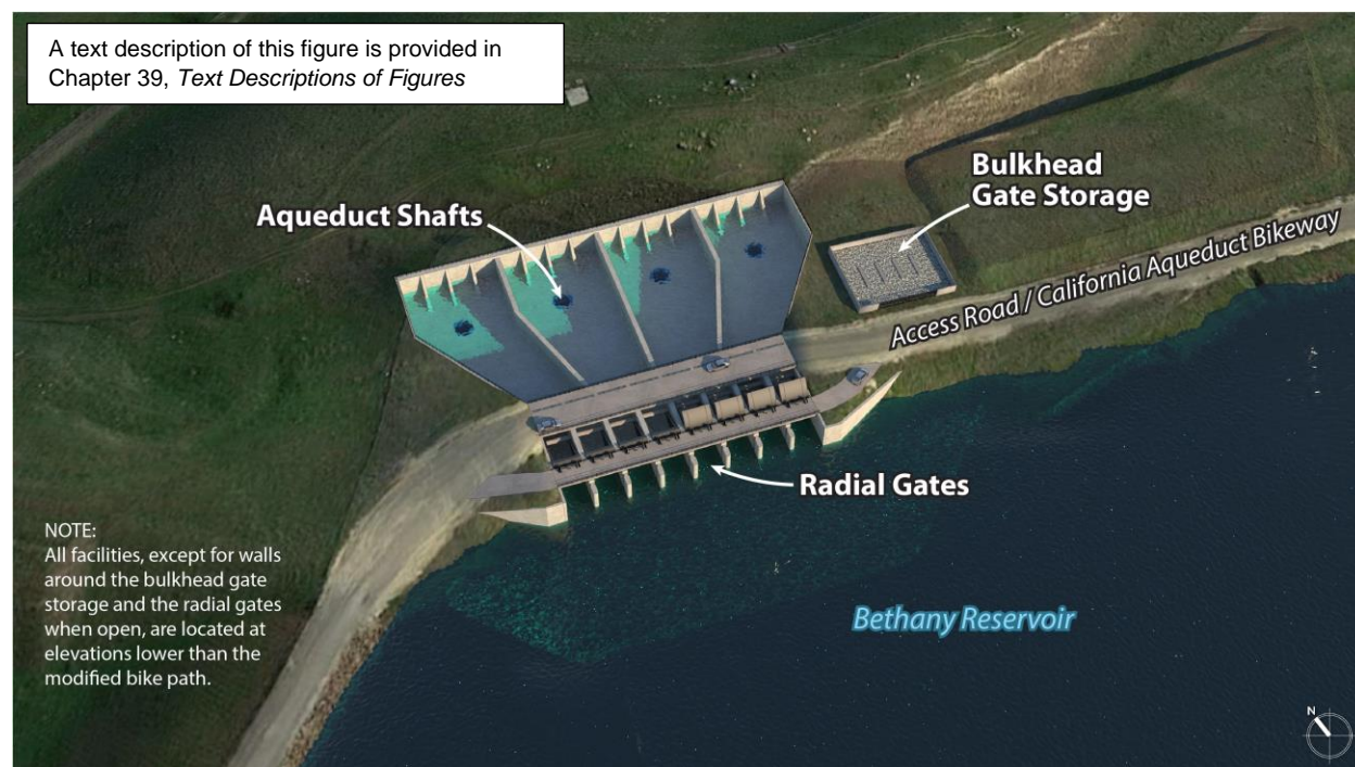
4 5 Figure 3-34. Bethany Reservoir Discharge Structure
